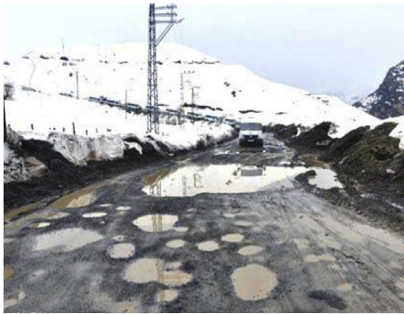
c) Cuts in road due to water, (Haberler, 2014)
