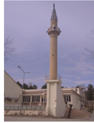
Fig. 2. Minaret of Firat University Engineering Campus Mosque
