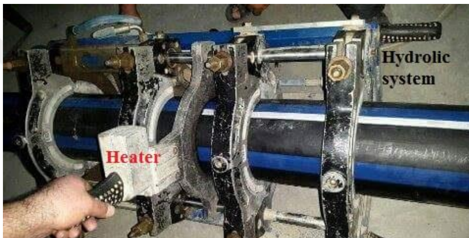
Figure 5.3. Heat saturation during putt the heater and adding pressure.
